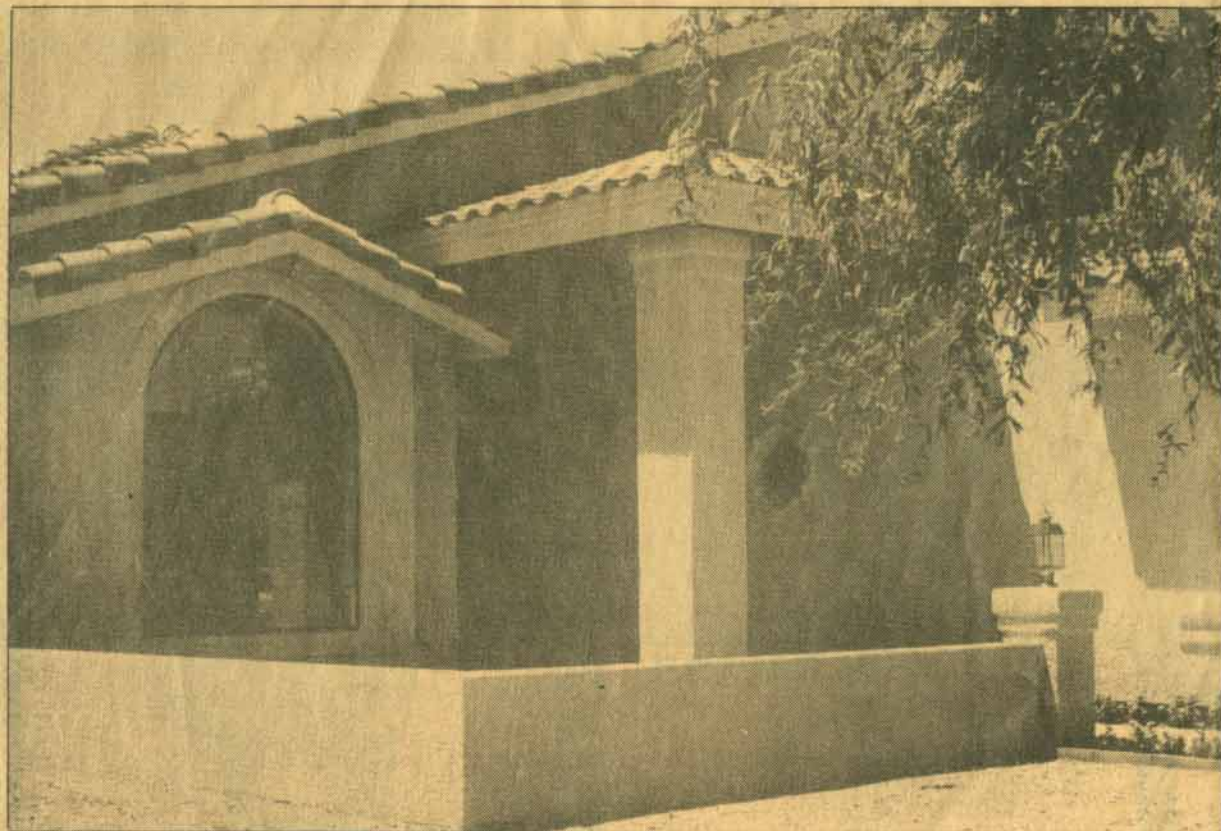
WELCOME HOME — Appealing entry to the new Nogales home of the Blain Tucker family is formed by the complementary
